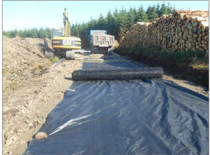
Figure 5: Crushed Rock Track build-up with Geotextile
