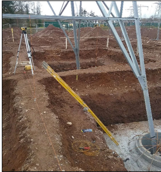
Figure 2: Stepped Back Excavation
